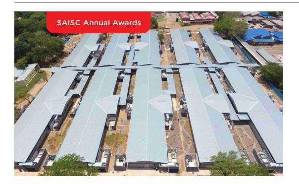
Steel was used in the construction of the Jubilee field hospital due to the light steel framing (LSF) and speedy construction methodology. Installation of the LSF walls were quick and easy and needed no cutting and chasing.
