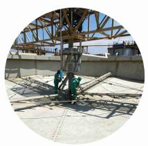
plant and the piping support system. A total of 85% of the piping was HDPE (high-density polyethylene), which needed several structural supports incorporated whilst keeping weights to a minimum and ensuring an aesthetically-pleasing final plant layout.
