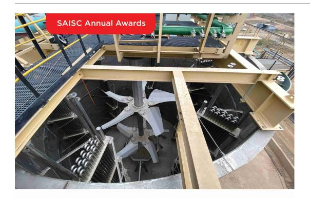
This technically challenging structural framing project entailed detailing, fabricating and constructing a gold-processing Biox plant. The primary objective thereof was to provide access to the various areas of the Biox plant and its piping support system.
