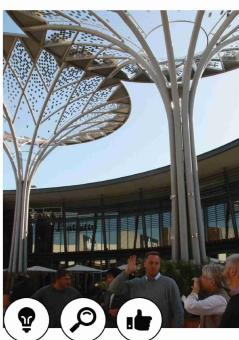
Three solar trees were designed to provide shade during the day, illuminate the space at night and harness renewable solar energy as a grid-independent power source.
