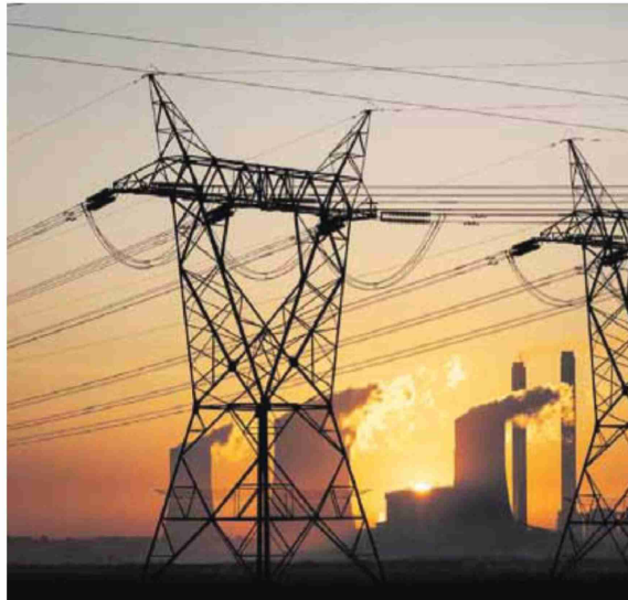
The sun rises behind Eskom's Lethabo coal-fired power station in the Free State in April, the month after the new Minister of Electricity, Kgosiensho Ramokgopa, was appointed. Energy experts disagree about whether his efforts will bring about a new dawn for South Africa's faltering electricity supply. Photo: Kim Ludbrook/EPA-EFE
